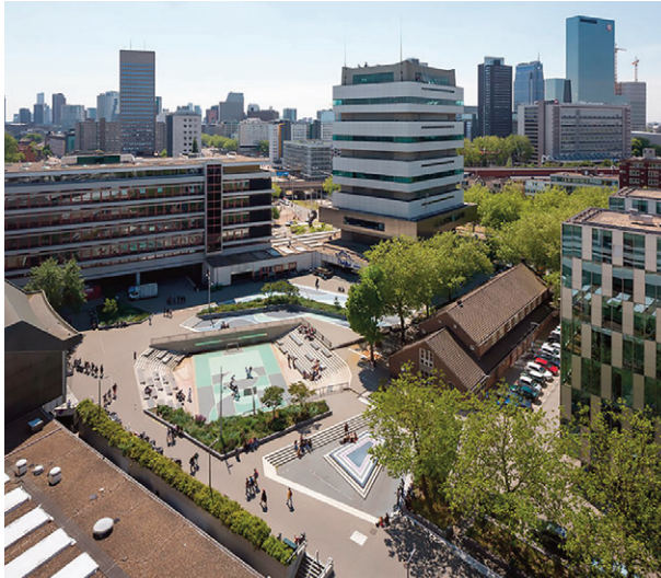
Fig. 12 | Watersquare in Rotterdam by De Urbanisten (credit: De Urbanisten).
