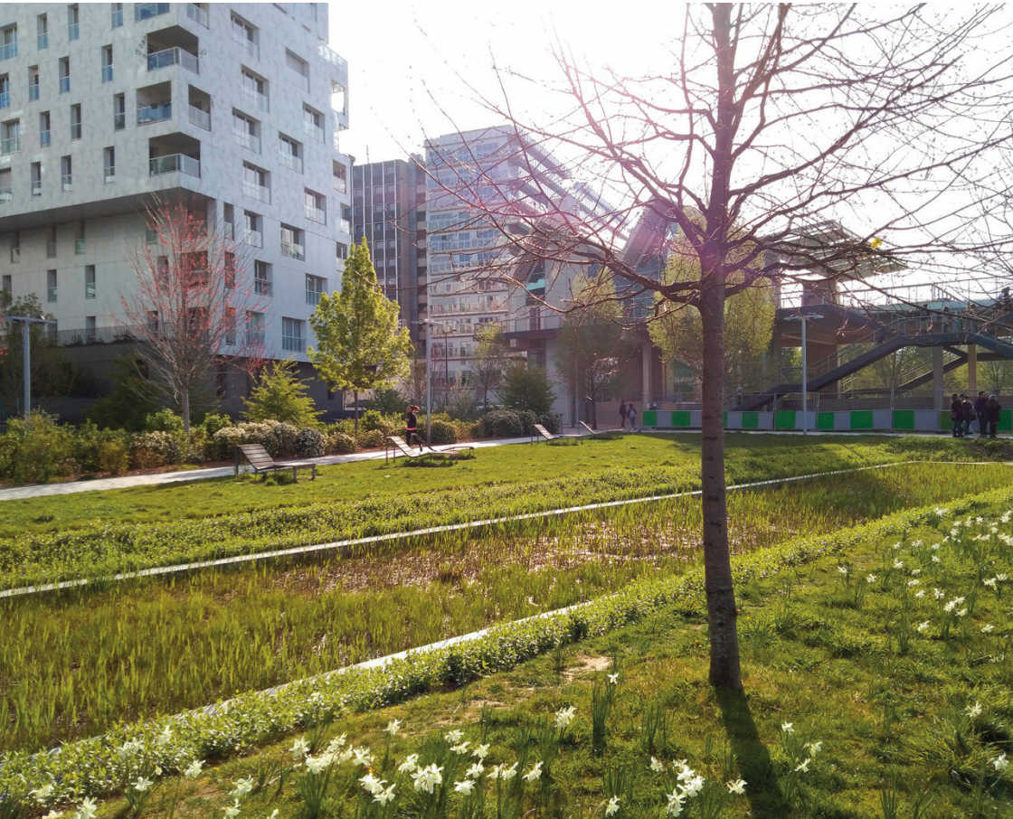
Fig. 1 | Clichy_Batignolles, Paris: View of the district's park area, detail of the rainwater harvesting basin, with attention to maintaining biodiversity (credit: M. Mariani, 2019).
