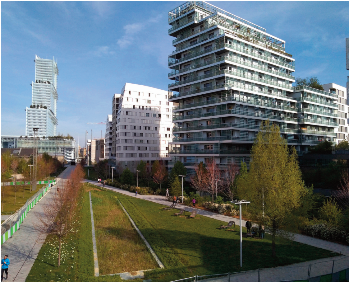
Fig. 2 | Clichy_Batignolles, Paris: View of part of the park and energy-efficient residential buildings. In the background, the building of the Palace of Justice by Renzo Piano (credit: M. Mariani, 2019).
