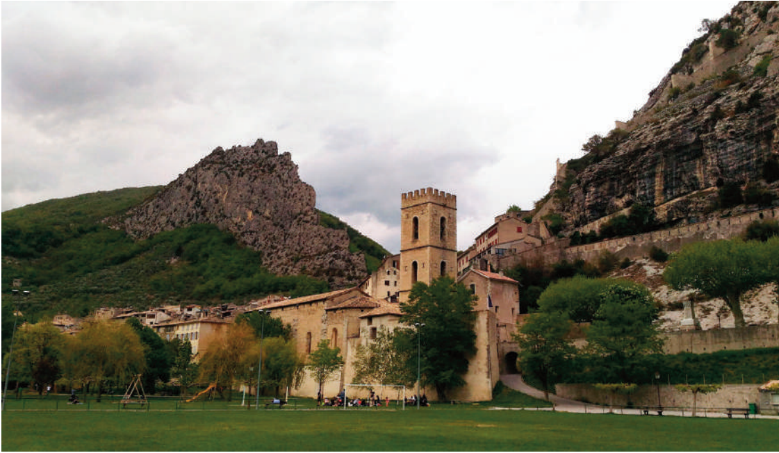
Fig. 4 | The small medieval center of Entrevaux, Provence France (credit: B. Di Palma, 2018).
