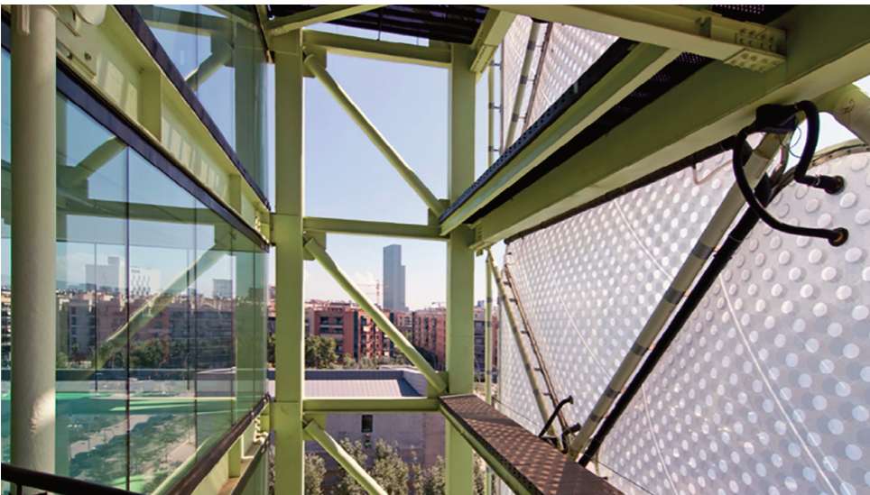
Fig. 3, 4 | Media ICT in Barcelona by Enric Ruiz Geli Architect and Cloud 9, 2010. The envelope is characterized by a counter-facade in EteFte (Ethylene tetrafluoro-ethylene), which, being able to be blown with air and nitrogen, becomes inflatable or deflatable according to the environmental stresses external (credit: Cloud 9).
