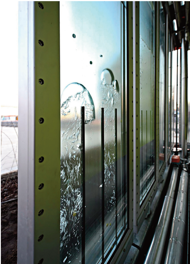
Fig. 1, 2 | Smart Material House BIQ in Hamburg by Splitterwerk Architects and Arup, 2013. The most significant element is the integration, on the south-east and south-west building façades, of flat-screen bioreactors, made up of microalgae (source: syndebio.com/).
