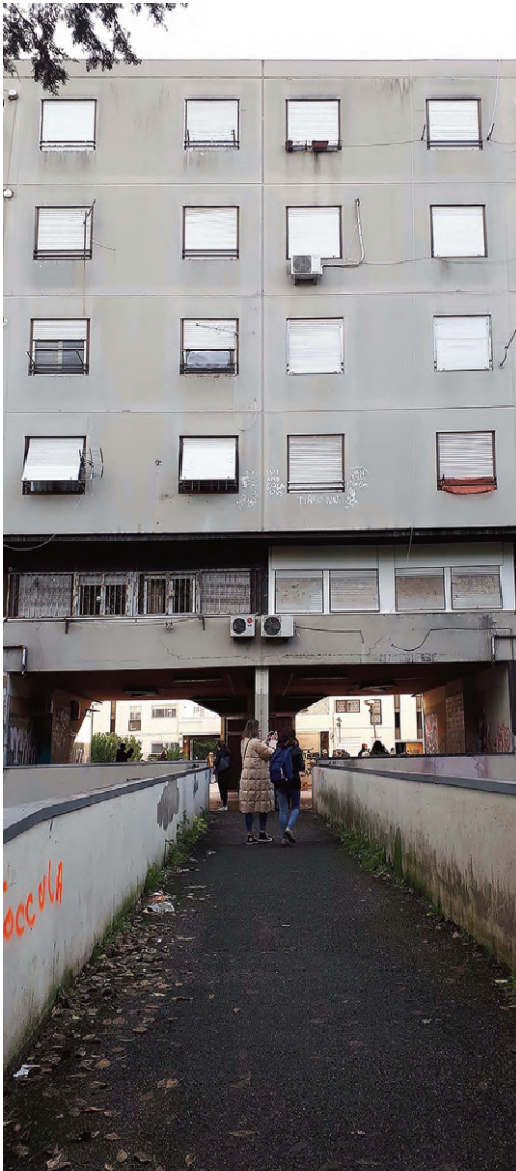
Fig. 3, 4 | Prefabricated sandwich panels façade and corner solution of the residential complex (credits: I. Coletta, 2020).
