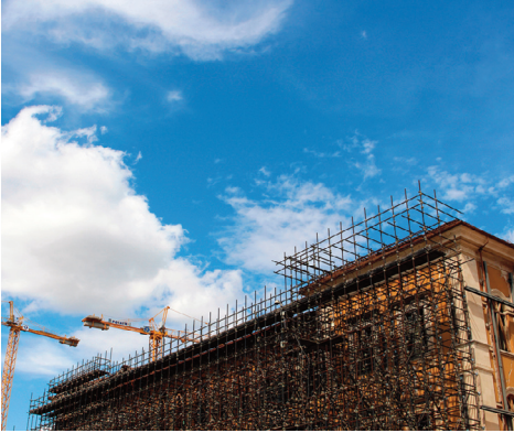
Fig. 13 | Protective structures outside 'E. De Amicis' Primary School in L'Aquila. Its full heavy temporary preservation occurred as per the normative framework – besides the extreme damages suffered after the 2009 earthquake – and lasted unmodified for almost a decade after the event (credit: photo of the Author, 2018).
