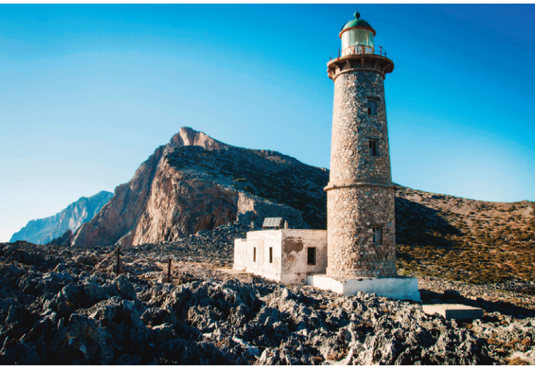
Fig. 5 | Antikythera: View of the lighthouse (1926) on the southern coast of the island (credit: N. Patsiouris).
